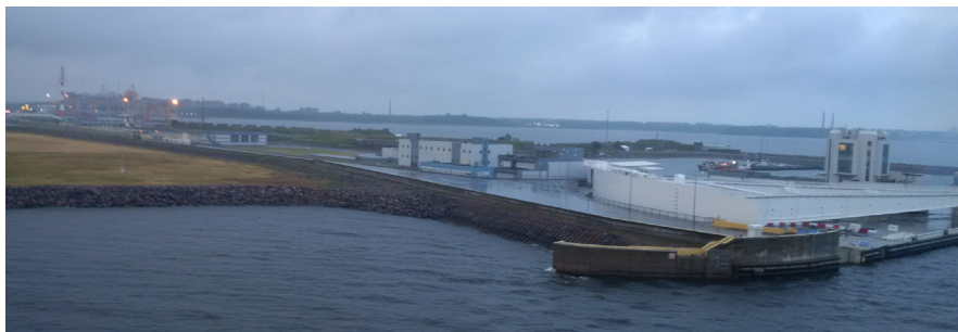
Passing through the S-1 gap in the tidal barrier that crosses the Gulf of Finland
